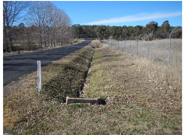
▲ Photograph 16: The southern drainage channel of Mann Street.
