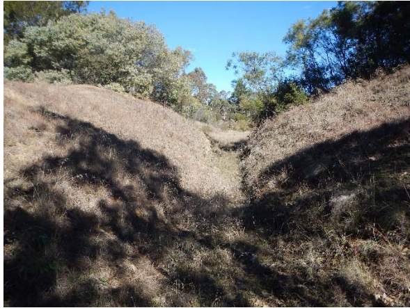
▲ Photograph 13: Drainage line from the skid pan in the south eastern corner.
