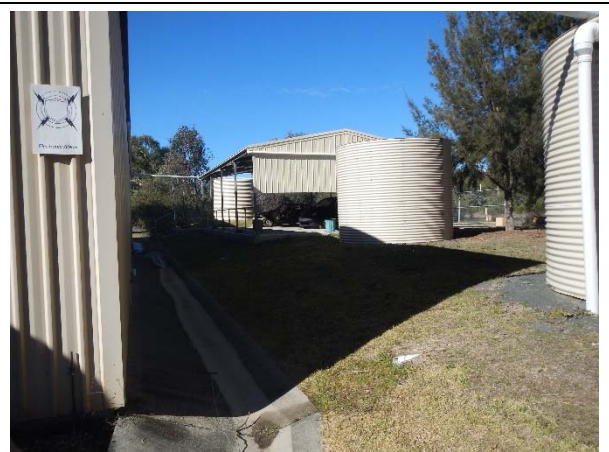
▲ Photograph 4: Mechanical area in the background with water collection tank in the mid and foreground. Concrete lined drainage channel.
