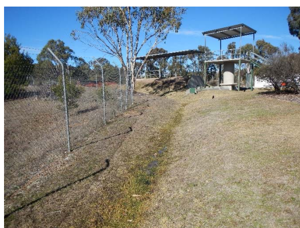
▲ Photograph 10: Surface water drainage line adjacent to boundary fencing.
