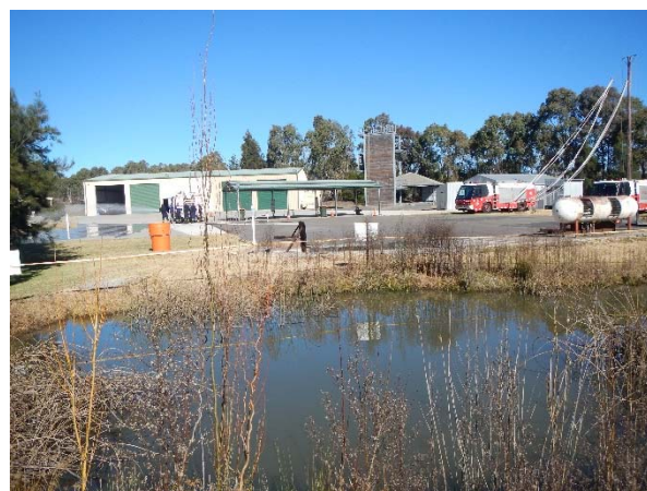
▲ Photograph 8: Facing south towards the main fire training area with the retention pond in the foreground..
