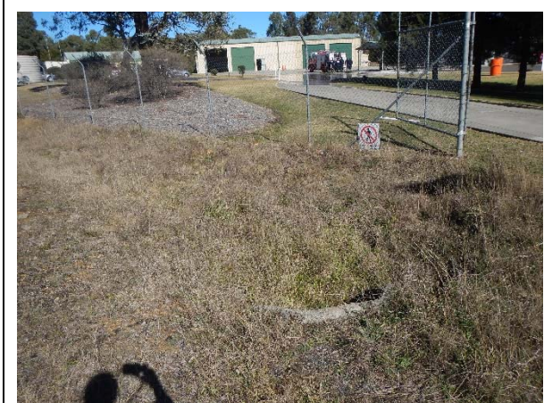
▲ Photograph 9: Culvert for surface water draining from the eastern area of the site.
